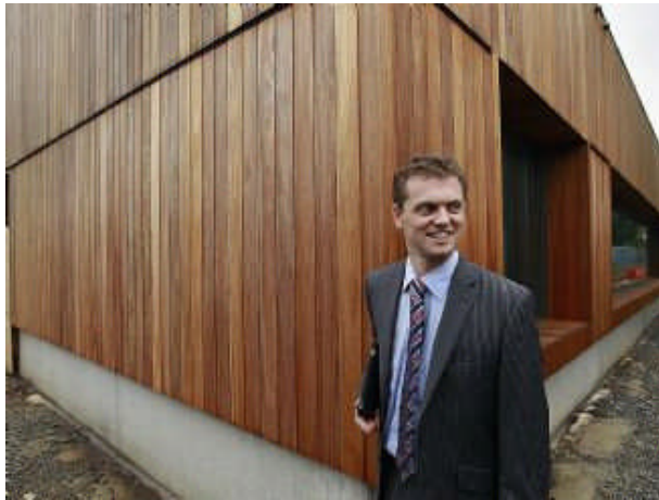
Dr Martin Preston inspecting work on Dandenong Hospital's new mental health building. Picture: Valeriu Campan
