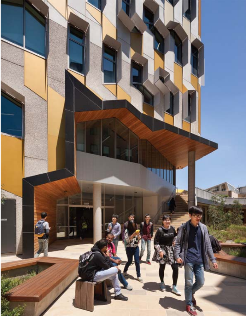
The north entry point invites users in with its angular entrance canopy
