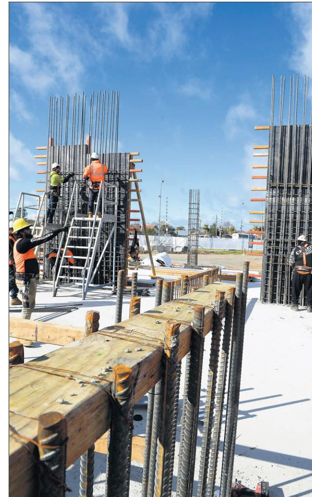
**In concrete:** Casings and steel cores for internal walls are being put in place.
