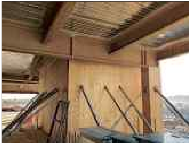
PRE-PREPARED: Some of the timber construction propped within the GovHub building. Most of the building is made off-site. Picture: Richard Nicholson.
