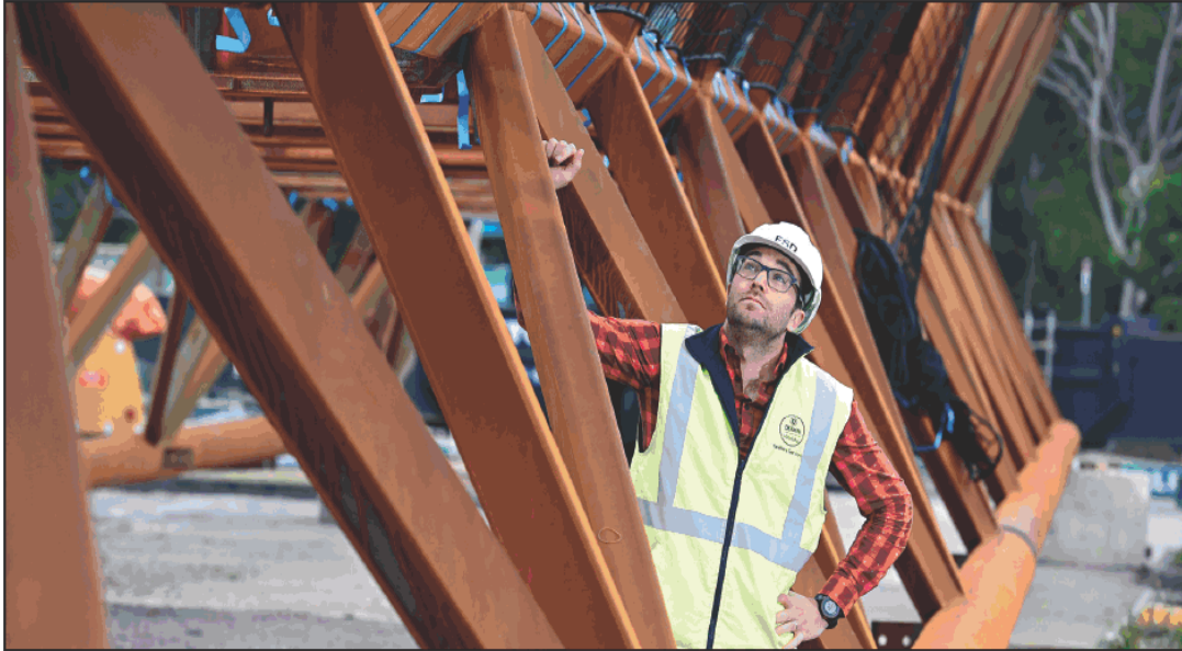
Project manager Mike David with the central truss of the Deakin University footbridge made from weathering steel that's designed to rust. Picture: LAWRENCE PINDER
