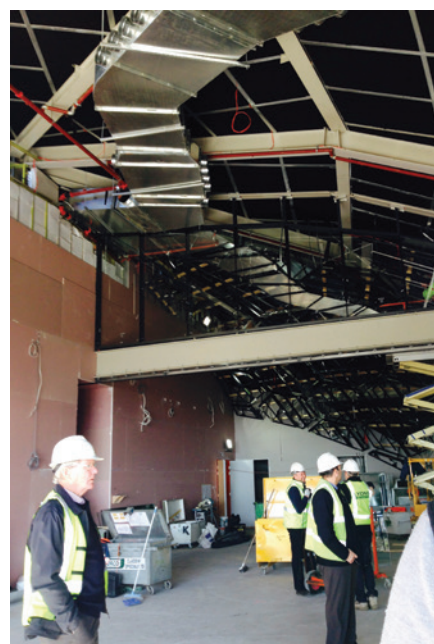
Inside the roof design.
