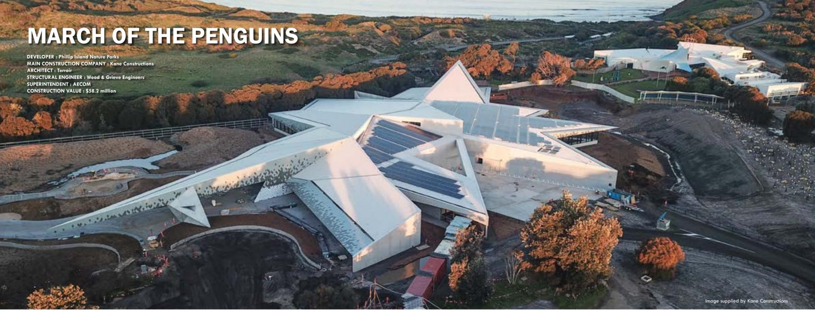
The \$58.2 million Penguin Parade Visitor Centre redevelopment has been designed with high levels of architectural finish including a complex roof and façade geometry comprising composite glue-laminated timber, steel and concrete with a zinc shingle façade.
